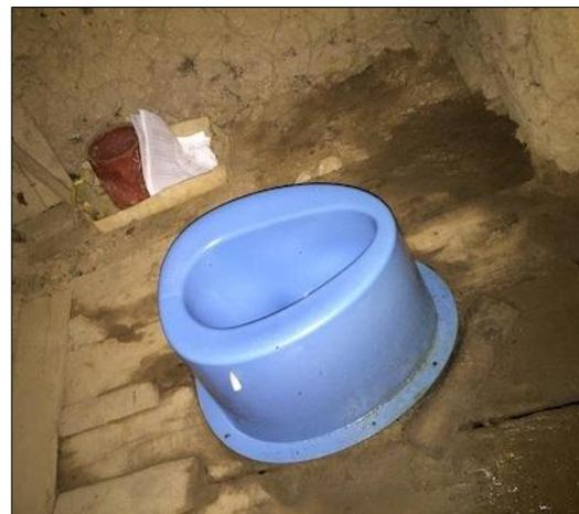
This SaTo toilet stool, shown here installed in Rwanda, offers a seated sanitation solution. It can be flushed using as little as 200 mL (approx. 6 oz.). Alternately, a pull-cord can be used to manually operate the trap-door flushing mechanism.
