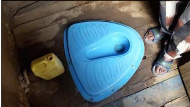
This bathroom in Rwanda showcases a slab-style SaTo pan that is an ideal solution for closing off open pit latrines from the open air. It operates with a trap-door mechanism that flushes with only 200 mL (approx. 6 oz.) of water, or can be activated manually using a pull-cord feature.
