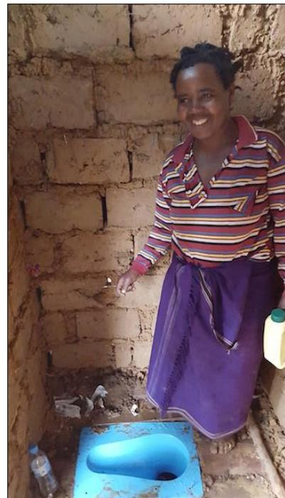
This adaptation of the original SaTo sanitary toilet pan now includes a wider flange. This feature facilitates installations into mud or wood floors, as pictured here in a bathroom in Rwanda.
